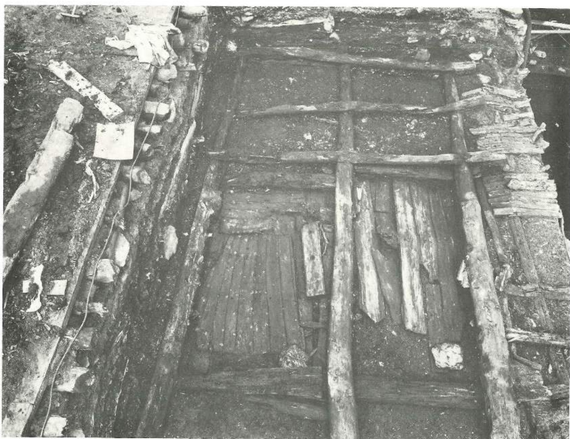
Fig 6-11 Fragments of ship's sides used in foundations
