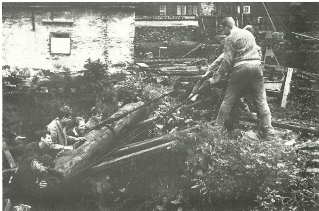
Fig 1-2 Many hands were needed to get the windlass from the "Big Ship" out of the excavation field
