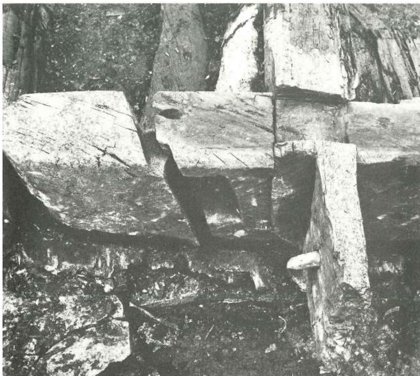
Fig 2-2 The large headbeam 90789 saw secondary use as a sill in a building
