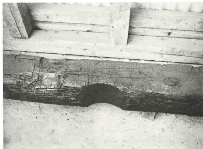
Fig 4-15 Detail of 90438 showing cutout for mast
