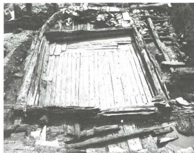
Fig 34 Ground-frame of Building 211 with intact floor, burnt in Fire V (1248). Looking south.
