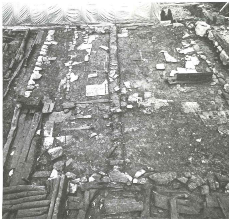
Fig 30 Building 20, burnt in Fire V (1248), with the remains of a stone-paved floor. Looking west.
