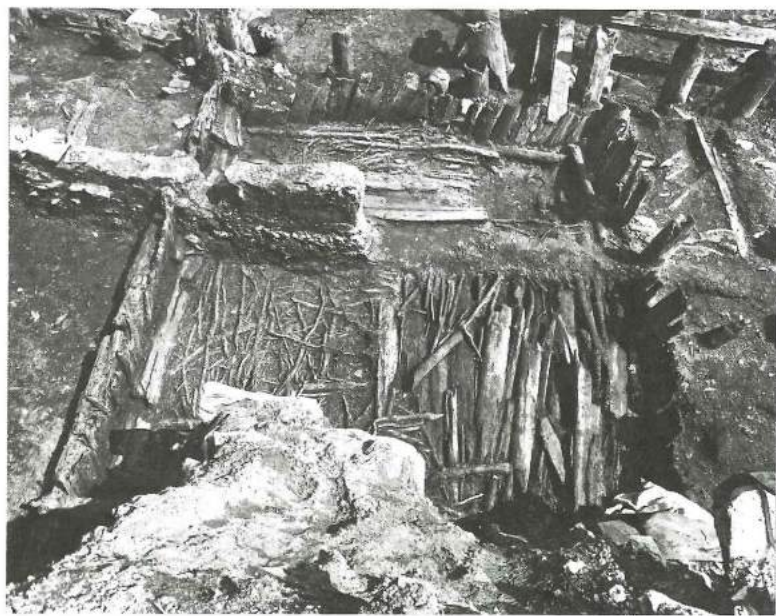
Fig 46 Building 38, with a vertical plank wall enclosing the area beneath the floor to form a cellar. The bottom of the cellar was covered with an "insulating" layer of old planks and branches. Burnt in Fire II (1170/71). Looking south.
