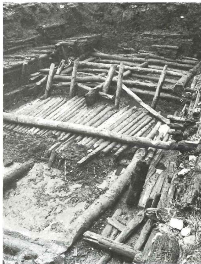
Fig 32 Logs placed close together over the foundation substructure Kar 117 in order to level up the surface. The posts of the contemporary quay can be seen in front. Period 4 (1198–1248). Seen from the north-east.
