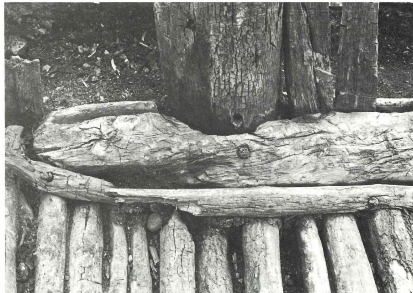
Fig 53 The third post from the west in the south wall of Building 45 with a hole for the wooden nail which can still be seen in the sill-beam, now lying below its original position. Looking south.
