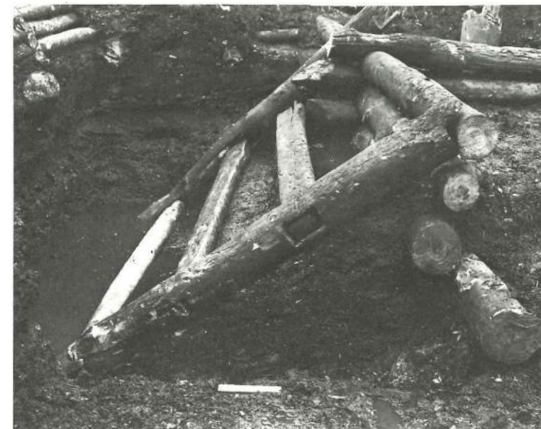
Fig 42 The strong, wide ladder found in front of the wharf (Kar 19) in Rows 5 and 6. Looking north.
