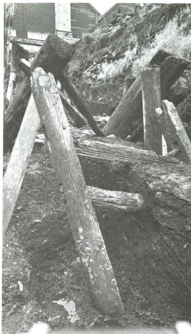
Fig 43 Remains of a ladder in front of the passage between Rows 1 and 2 in Period 2 (–1170/71). Looking east.
