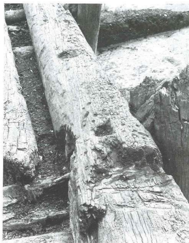
Fig. 79. Close-up of the horizontal beam at the front of the Søstergården South wharf at the beginning of Phase 3.2. It was embedded with stones to provide a better grip for the feet when embarking or disembarking.
