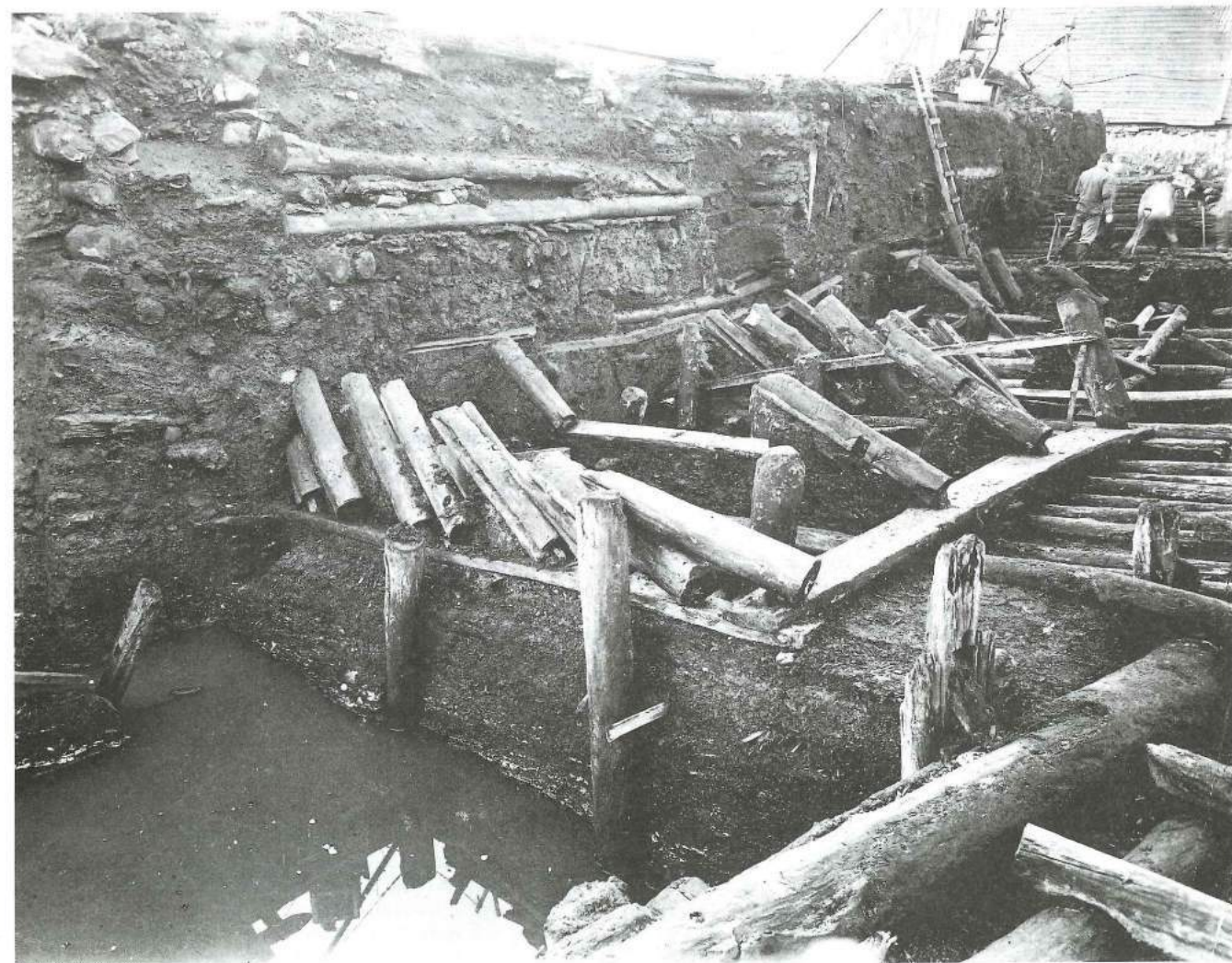
Fig. 72. Massive, well-preserved foundation posts, standing on sole-plates under Building 397 in Søstergården North, erected after 1332. Seen from the south-east.
