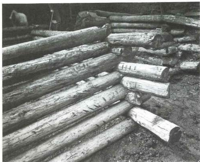
Fig. 51. Part of the Period 4 foundation substructure Kar 61 in Engelgården, seen from the south-east. The structure was prefabricated: the marks on the logs were for guidance when re-assembling it.
