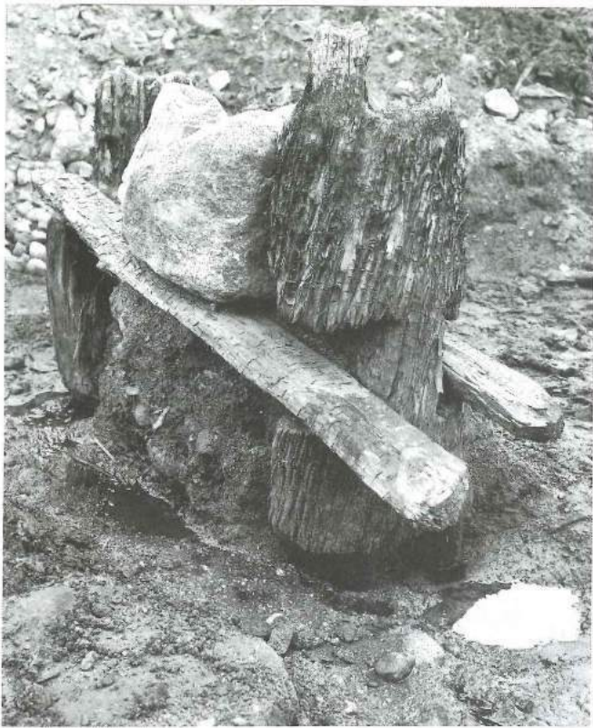
Fig. 89. Pair of foot-braced posts from a jetty at Borgund-kaupangen in the district of Sunnmøre.
