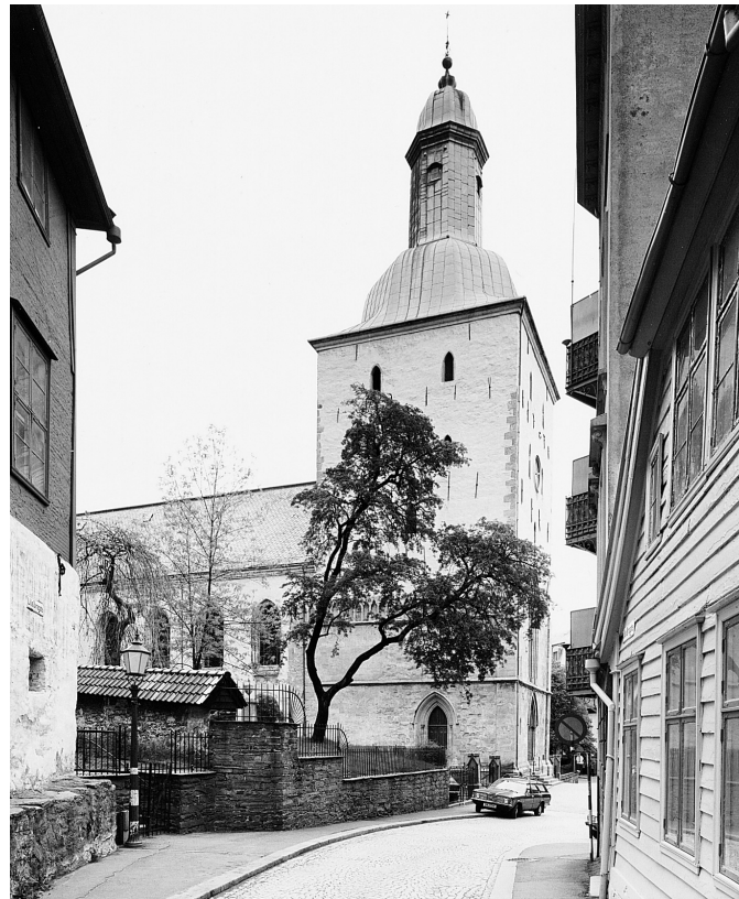
Fig. 13. St. Olaf's of the Franciscans. Most of St Olaf's of the Franciscans, the present-day Cathedral of Bergen, was rebuilt, as it is seen from the north today, after the fire of 1248, including the 'fore-hall' which is now the base of the early eighteenth-century tower. The priory which burnt in 1464 was situated south of the church.
