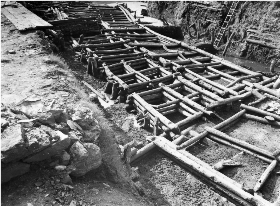
Figure 2.5 Caissons in the area of Gullskoen and the tenement Søstergården. From the Bryggen excavation 1955–1968. Photo: Bergen Museum.
